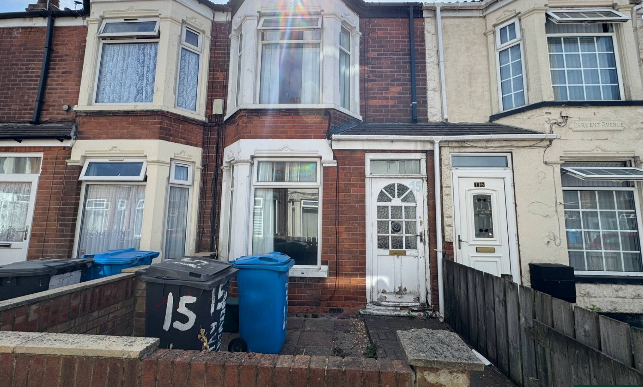
15 Derwent Avenue Hampshire Street, Hull £75,000
