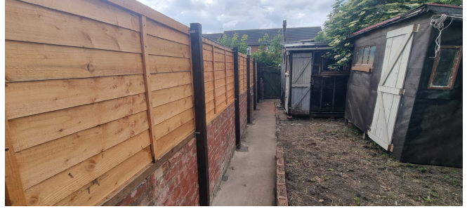
Rear garden / new fence
