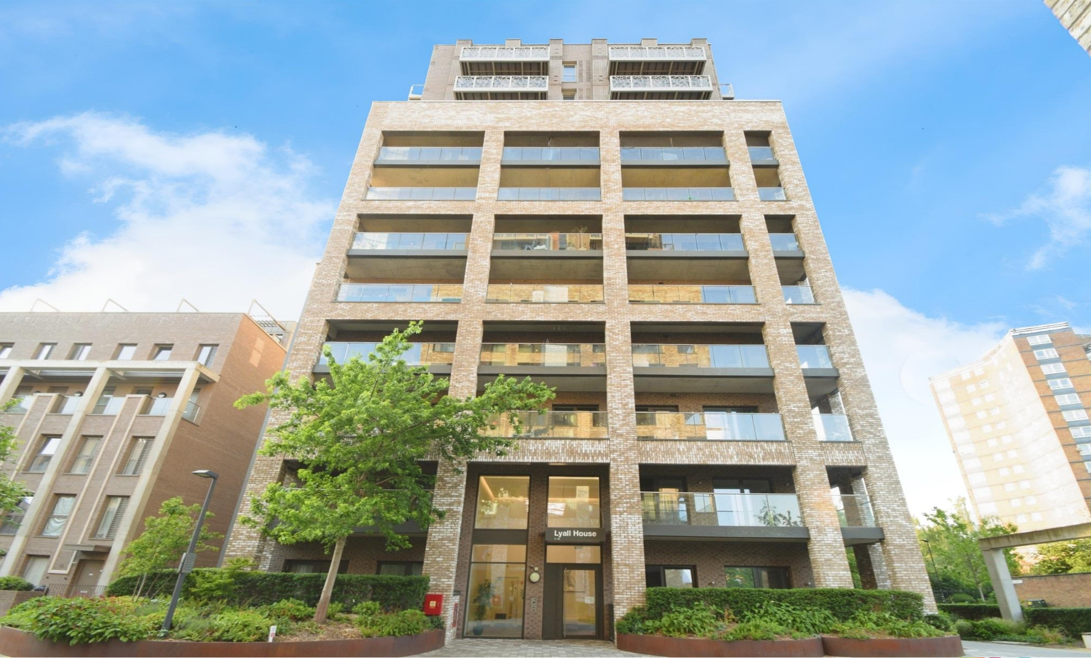
Lyll House, Shipbuilding Way, London, E13 9DW
