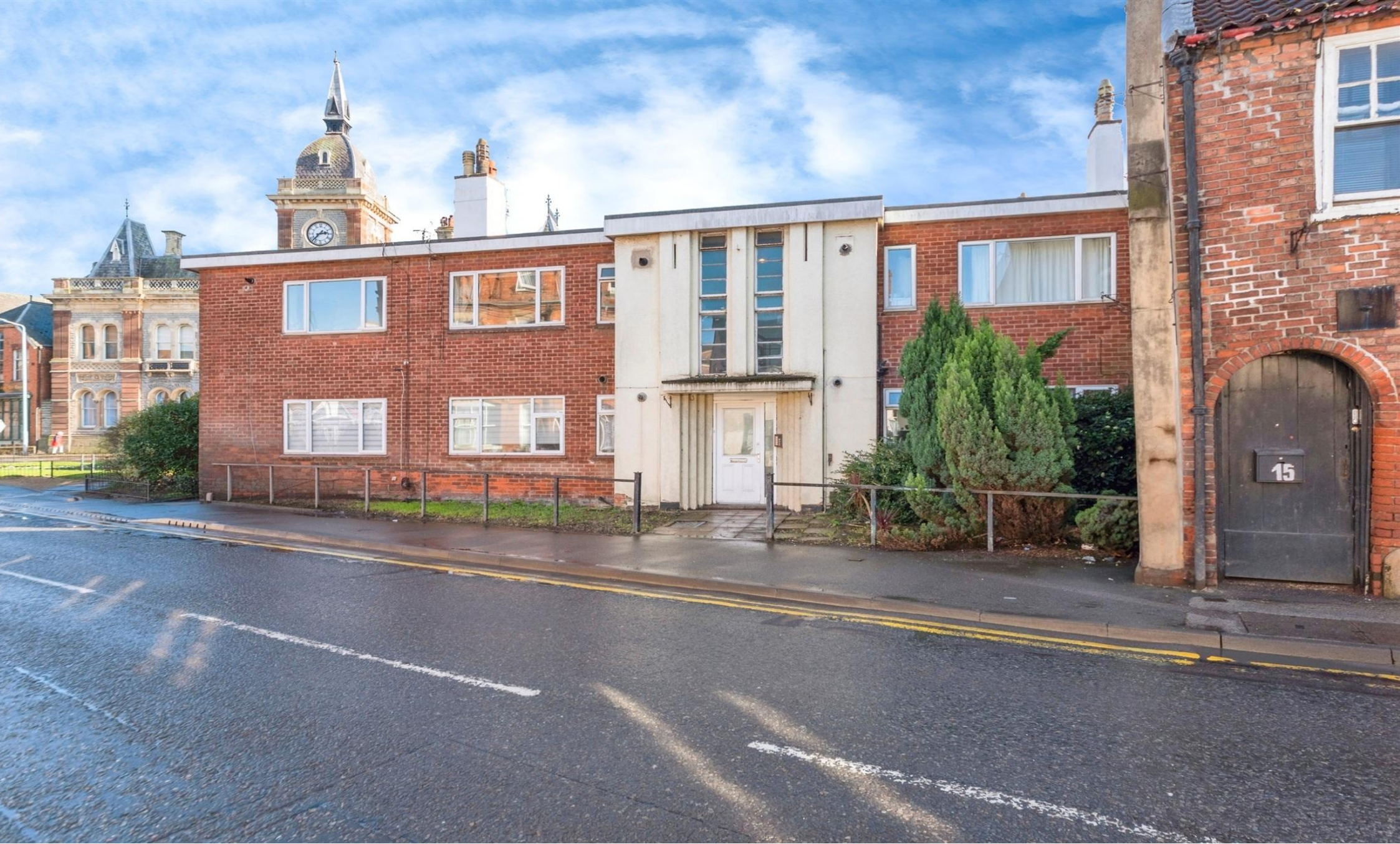
Portland Court, Newark NG24 4XQ
