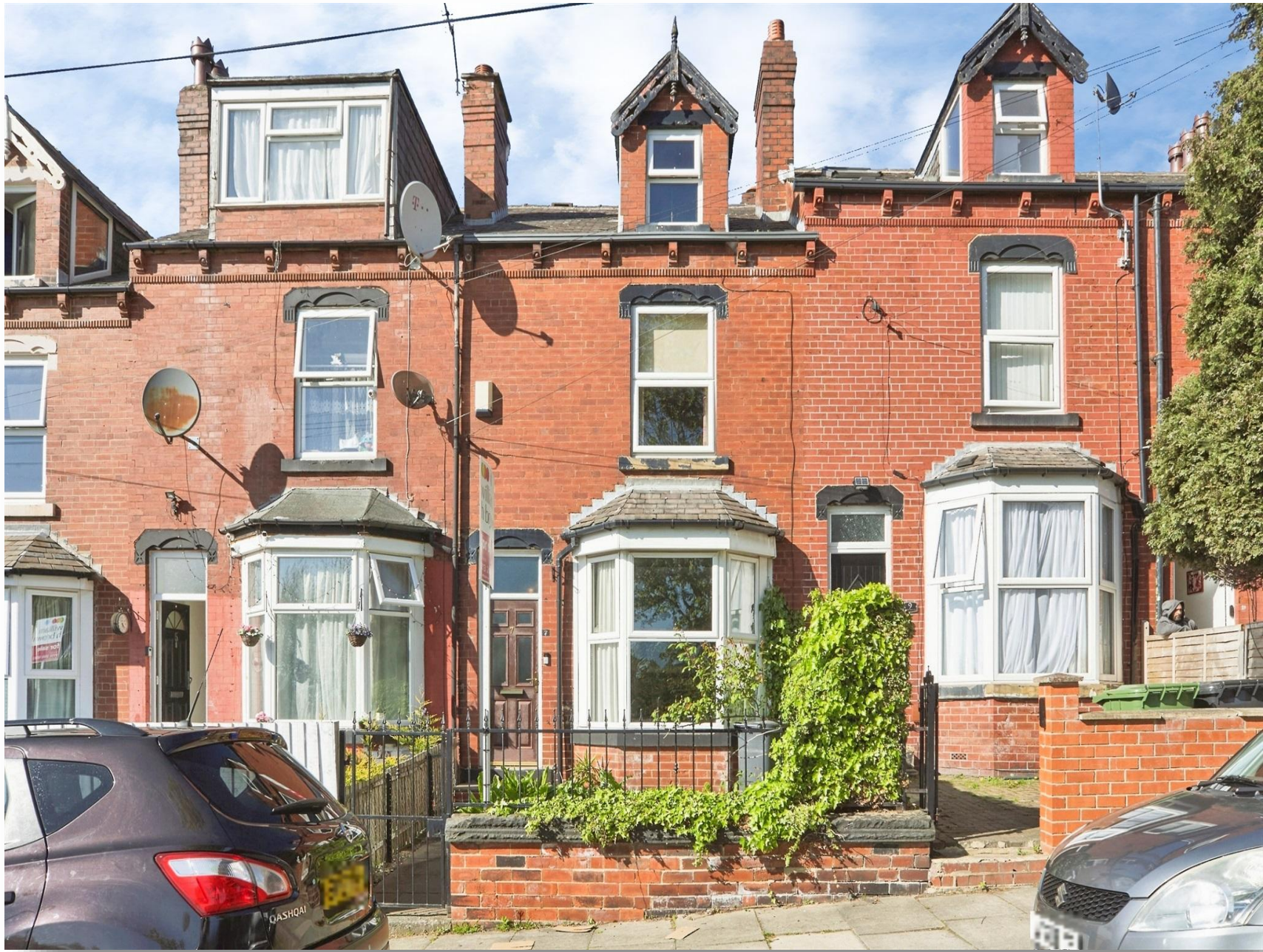
Banstead Terrace East, Leeds LS8 5PX
