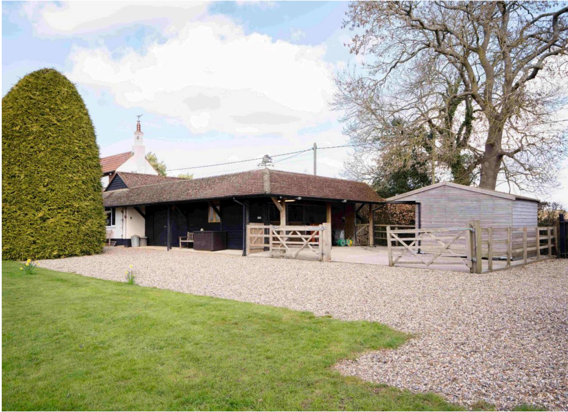
CORFIELD, ARREWIG LANE, CHESHAM
