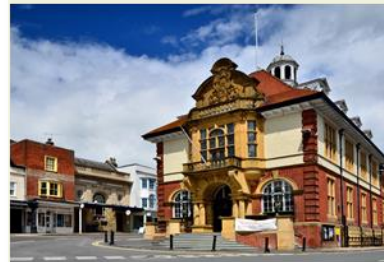
Marlborough Town Hall
