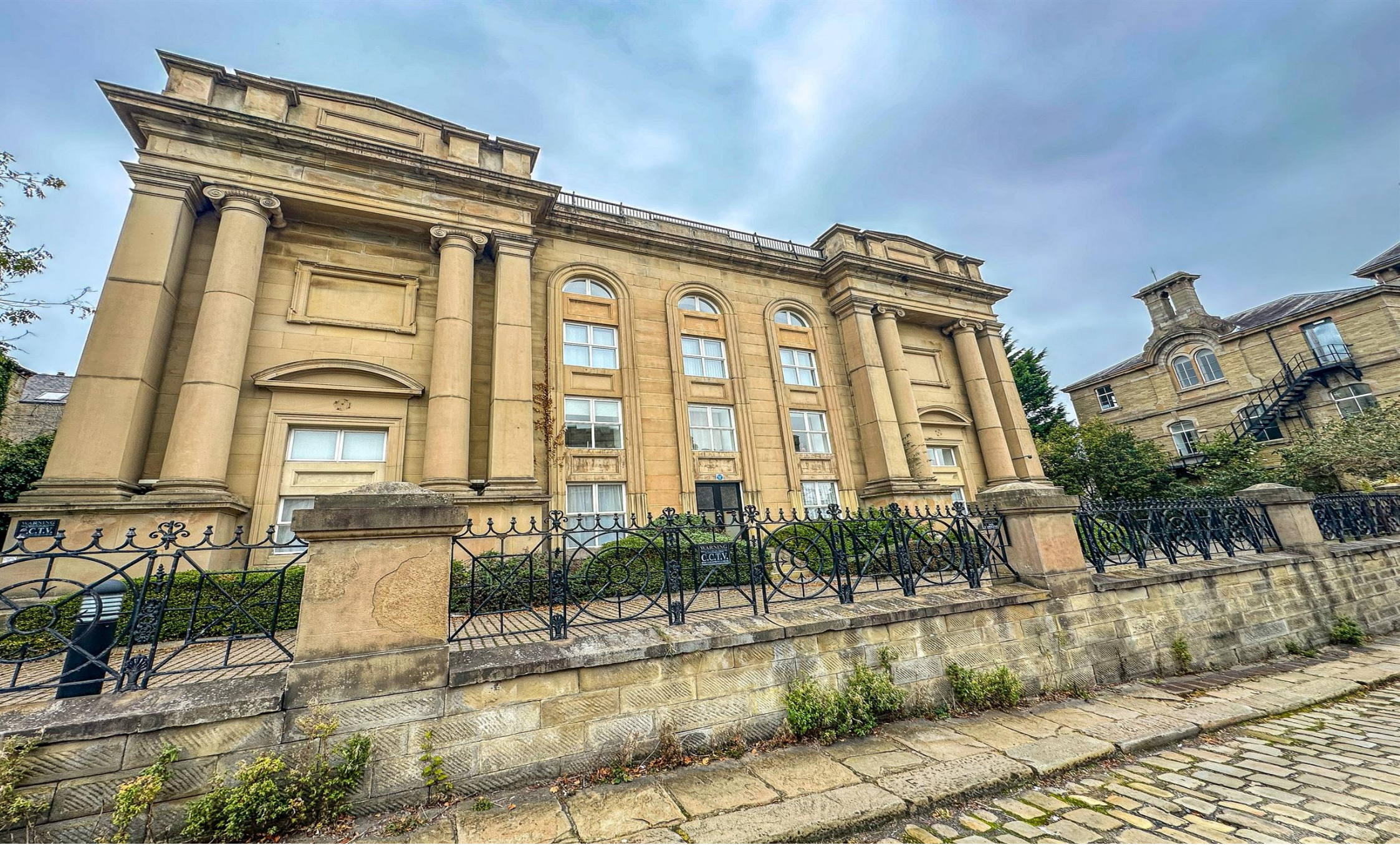
Highfields Court, Highfields Road, Huddersfield, HD1 5NG
