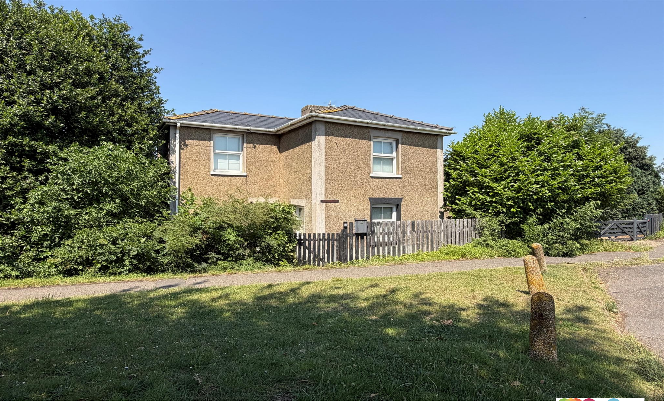
Bridge House East East Bank, Sutton Bridge Spalding PE12 9YN
