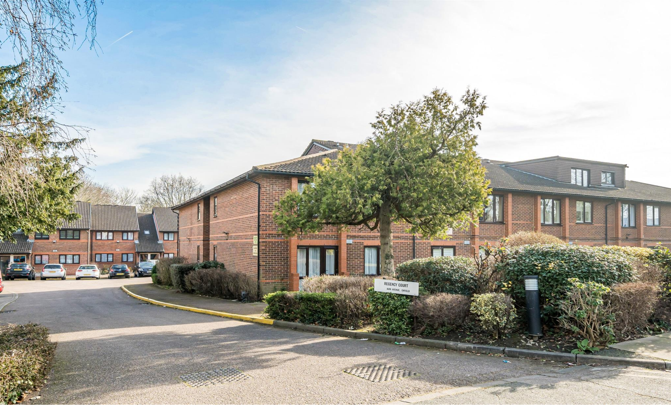
Regency Court, Park Avenue, Enfield, EN1 2HR
