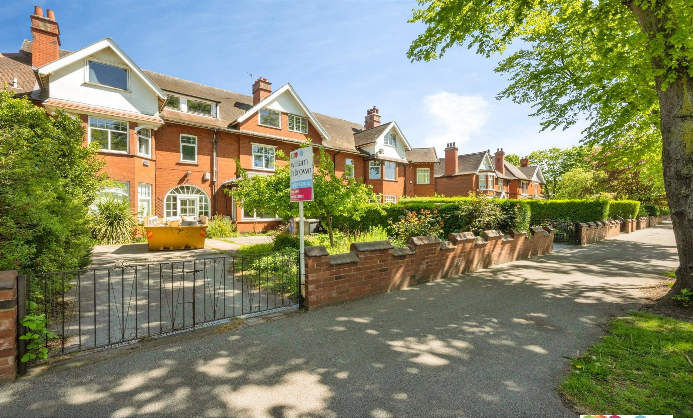
Town Moor Avenue, Town Moor Doncaster
