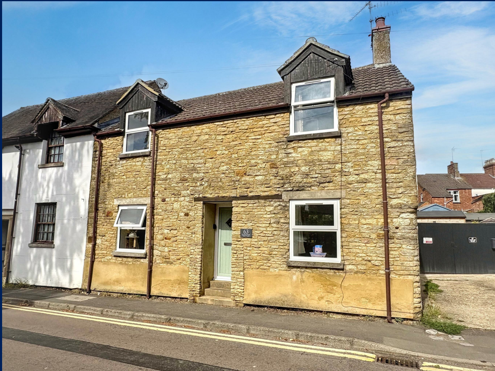
The Old Bakery, 63 London Road | Wollaston | NN29 7QP
