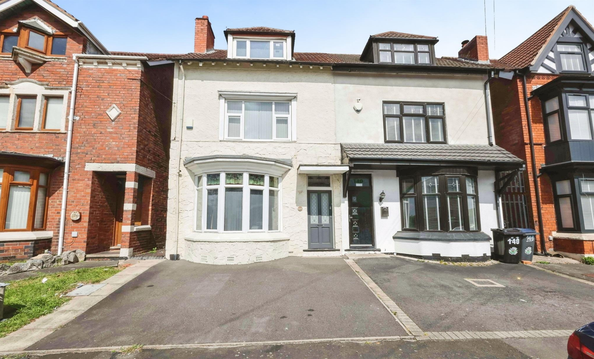
Manor Road, Stechford, Birmingham
