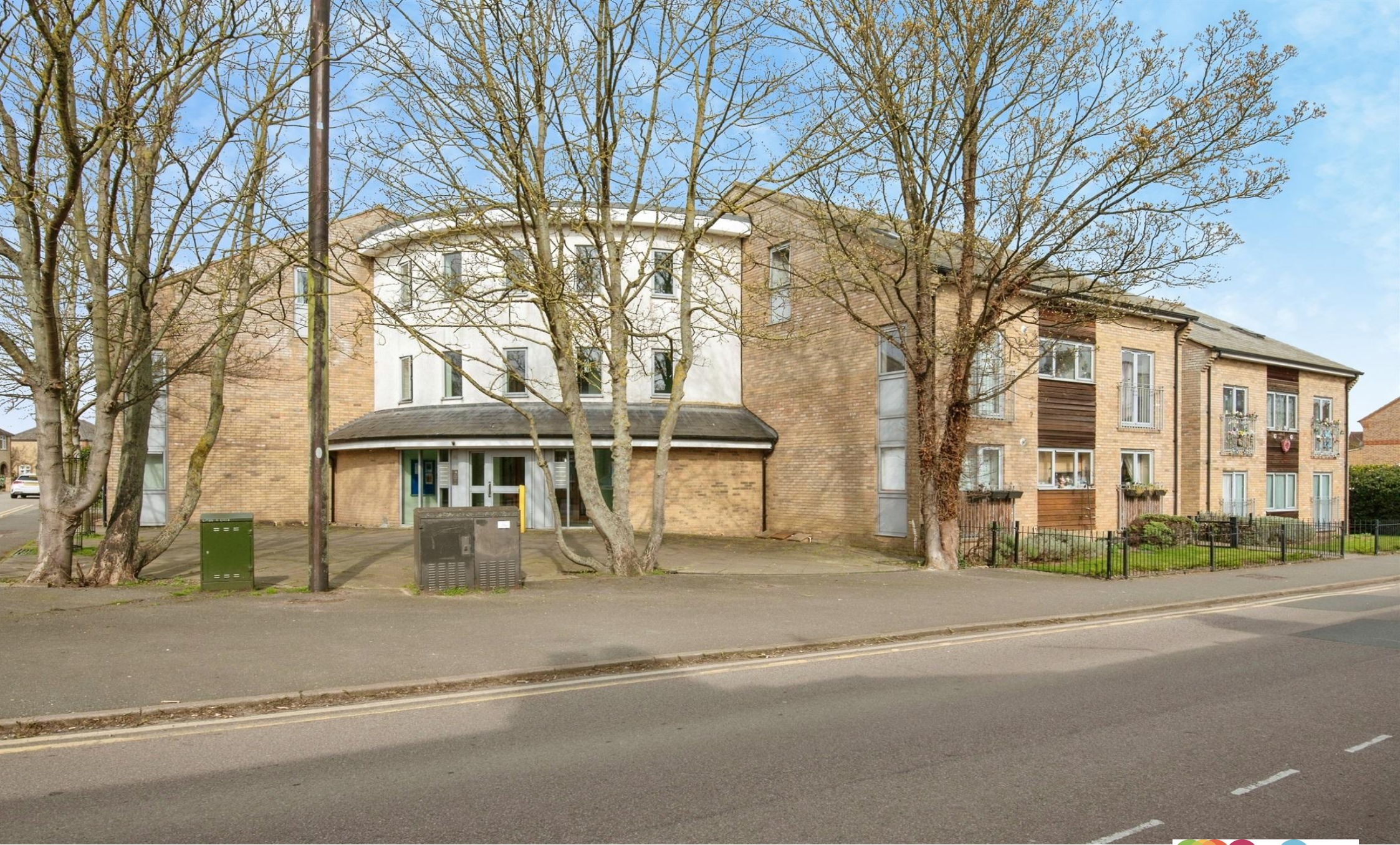
Cain Court, Victoria Crescent, Royston, SG8 7EW
