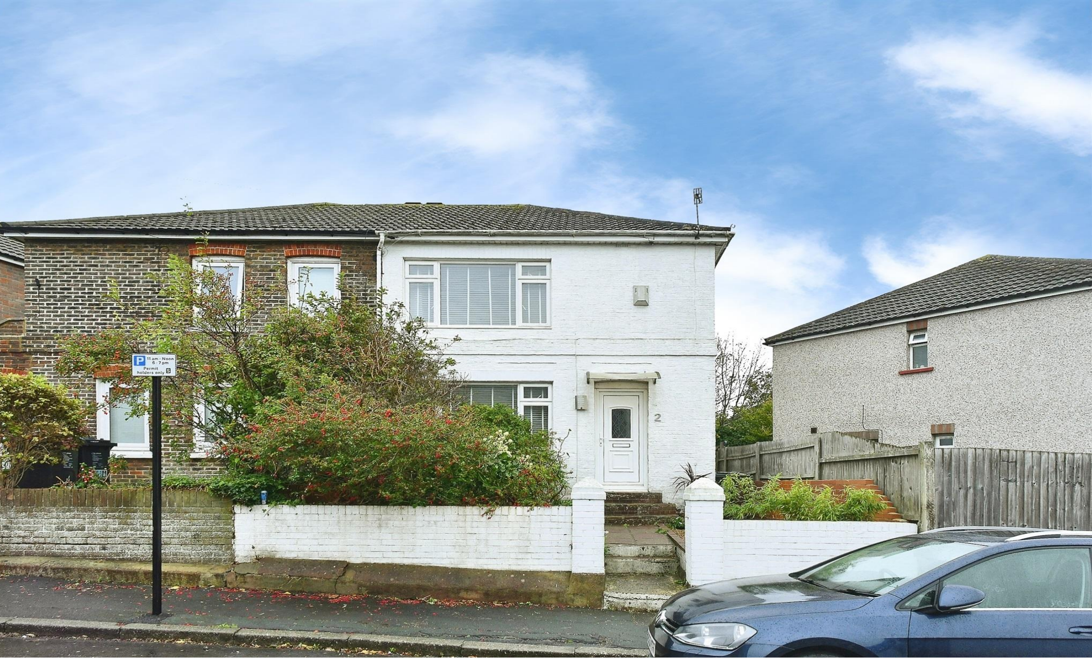
Plumpton Road, Brighton BN2 9YL
