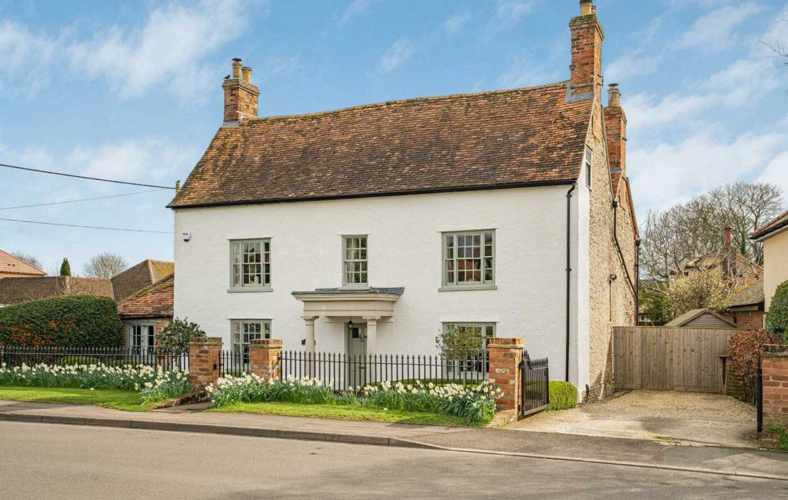
34 BROOK STREET, BENSON
