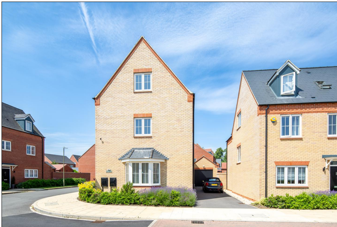
Garage and 2-3 Car Driveway
