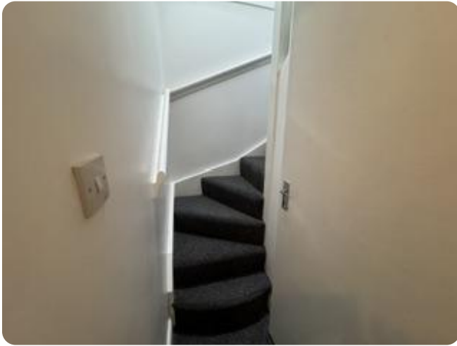
STAIRS TO LOFT
