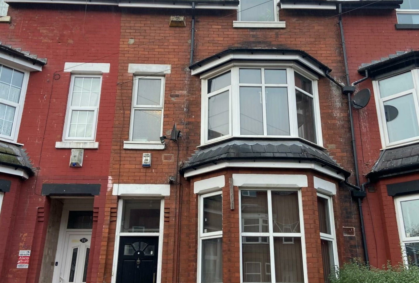
7 Bed House - Semi- Detached located in Fallowfield £4,060 PCM
