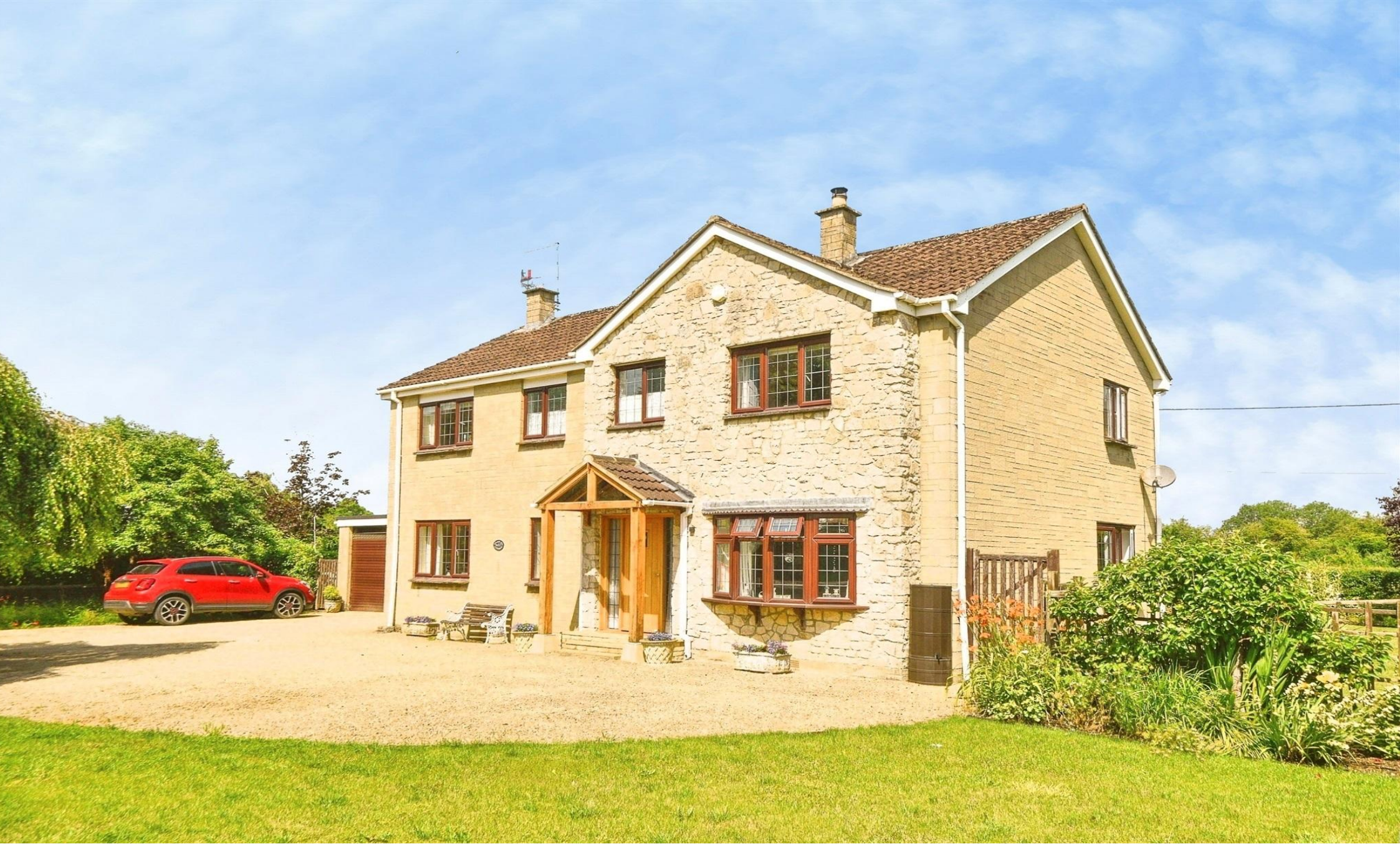
Bradley Cottage Main Road, Christian Malford, Chippenham, SN15 4BD
