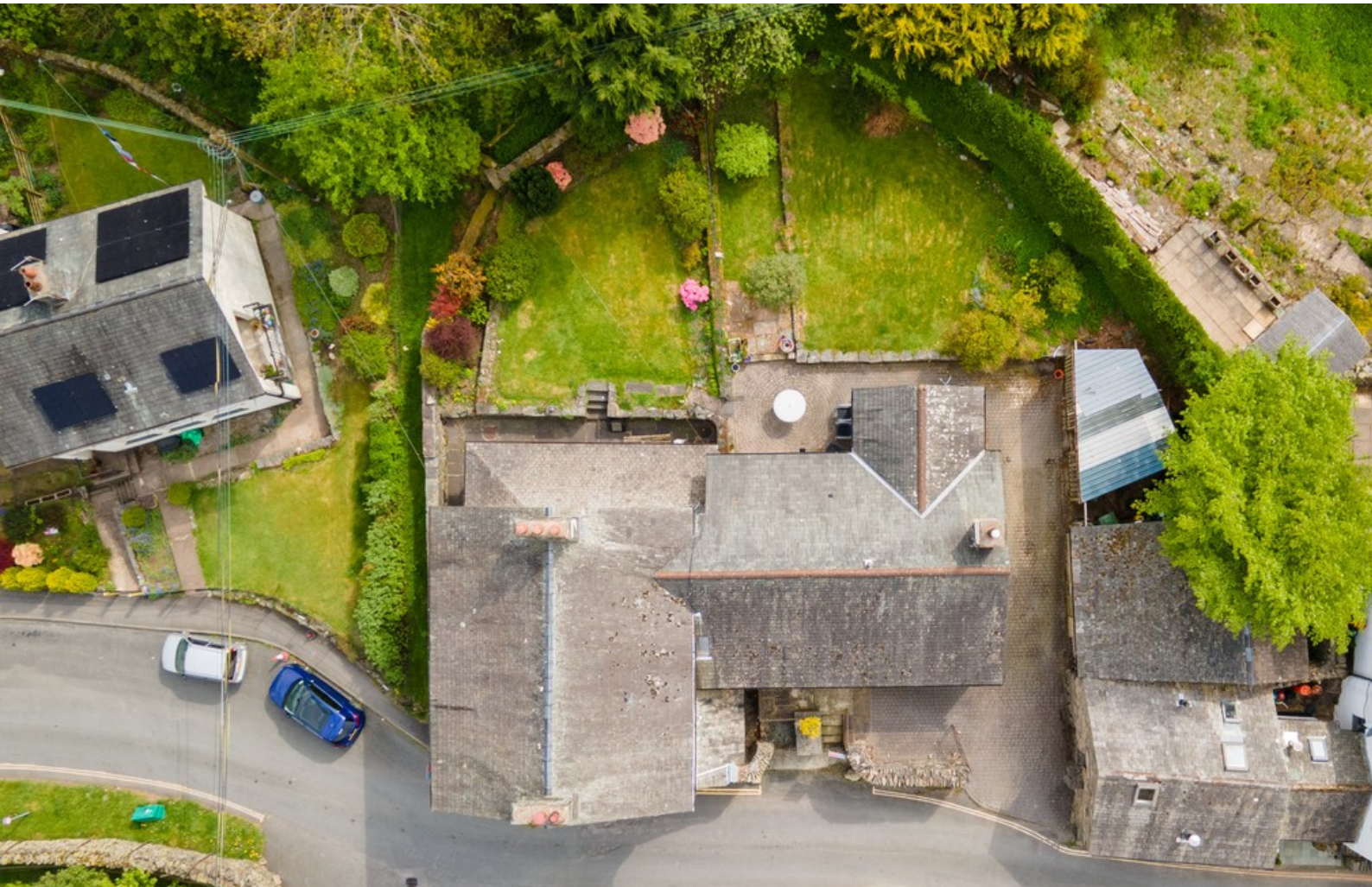
Aerial View of Cuthbert House & The Bungalow
