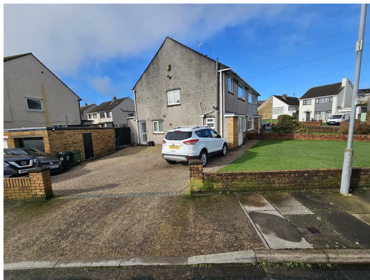
Rear Garden A small private garden with a paved patio area leading to an artificial lawn being enclosed by timber fencing
