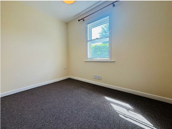
Triple glazed window, wall mounted electric heating radiator
