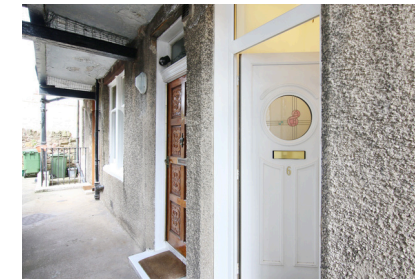
ENTRANCE VENNEL LEADING TO SHARED COURTYARD
