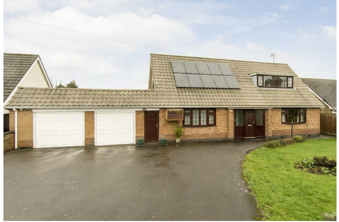
Double Garage 21'5" x 20'8" (6.53m x 6.30m)
