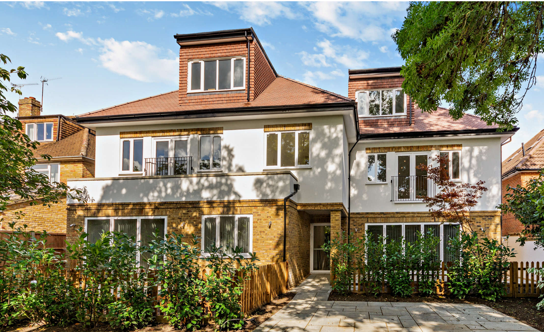
A one bedroom ground floor apartment Swakeleys Road, Ickenham, UB10 8DL
