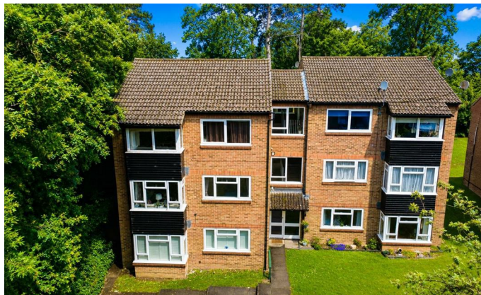
COMMUNAL ENTRY DOOR
