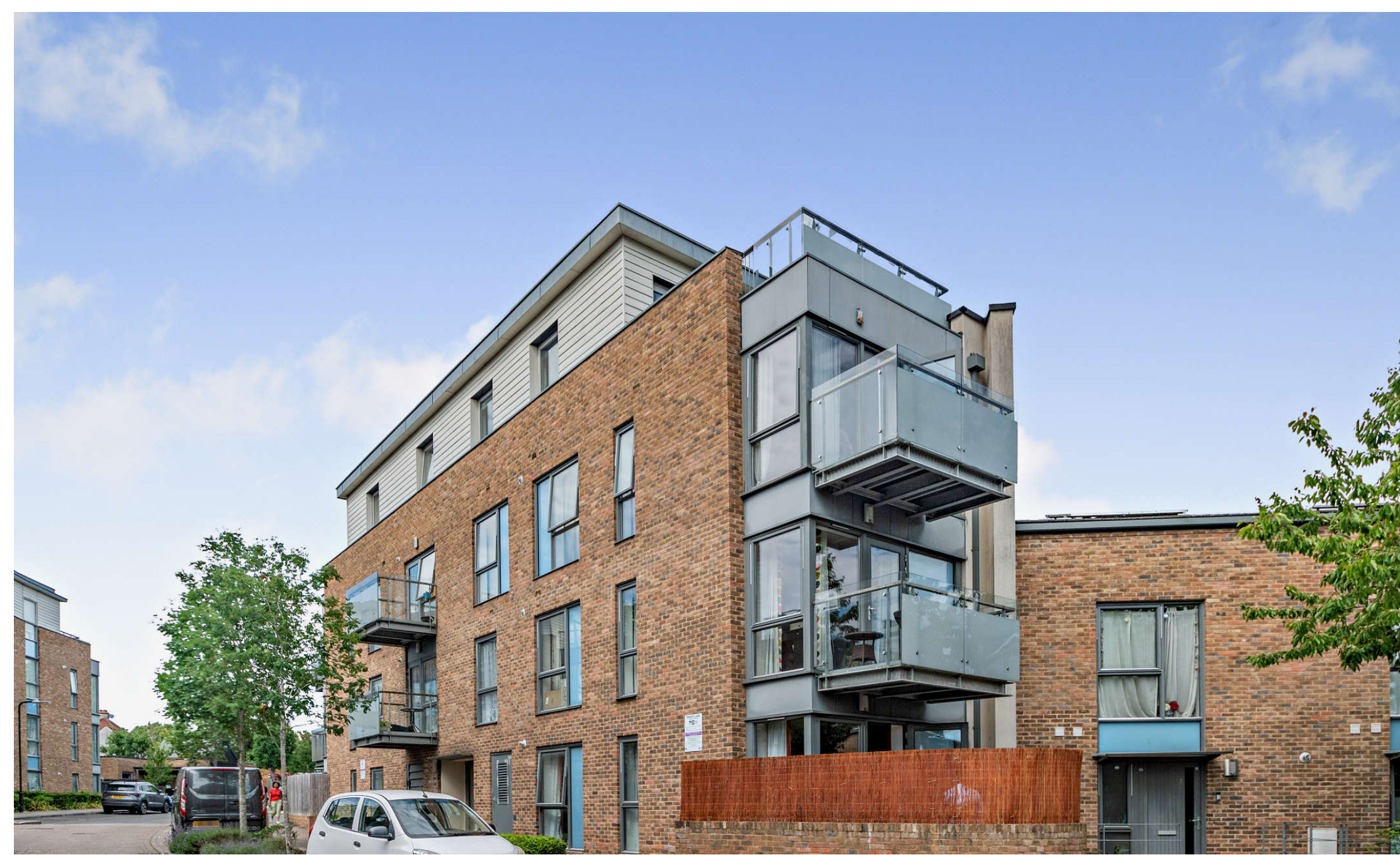
A two bedroom, two bathroom apartment with a balcony 2 Caulfield Gardens, Pinner, HA5 3AE
