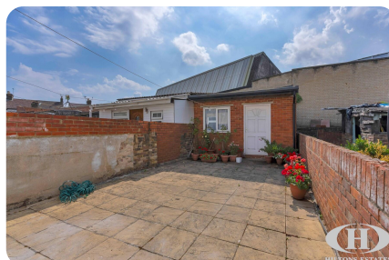
REAR PATIO & OUTBUILDING
