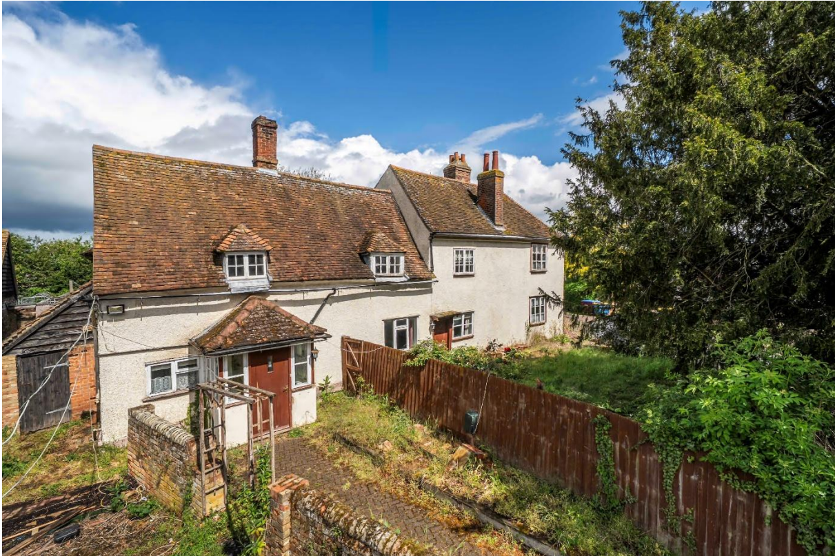
Village Farm, 4 St. Johns Road, Moggerhanger, Bedford, Bedfordshire MK44 3RJ
