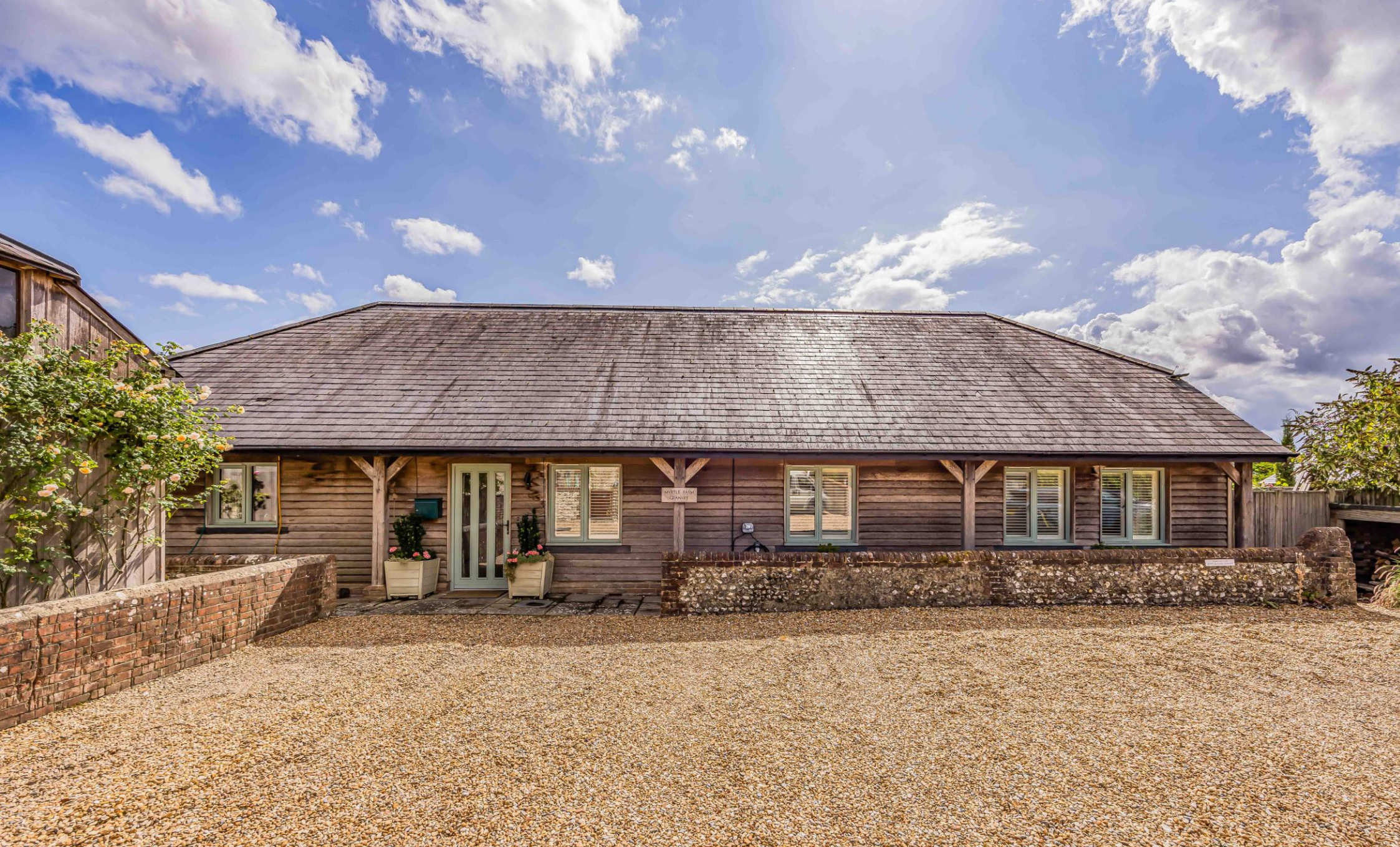
Myrtle Farm Granary, Blendworth Lane, Horndean, Waterlooville, Hampshire, PO8 0AA
