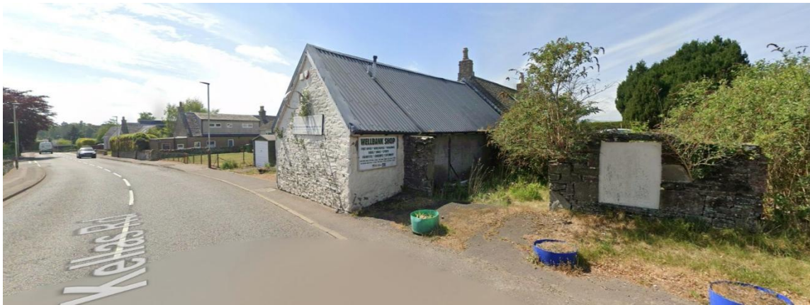
Above – North approach on Kellas Road. The rear garden area is heavily dilapidated, acting as an eyesore at present.
