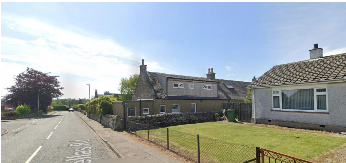
Above –Kellas Road, neighbouring property to the South demonstrates similar configuration and dormer placement to the proposals.
