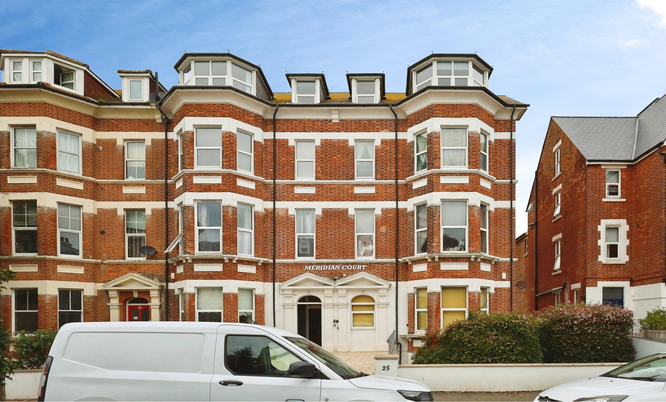
Meridian Court Jevington Gardens, Eastbourne BN21 4HR
