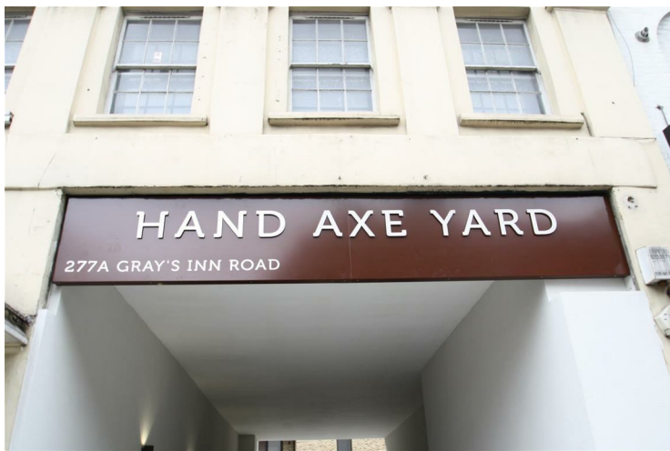
GRAYS INN ROAD ENTRANCE
