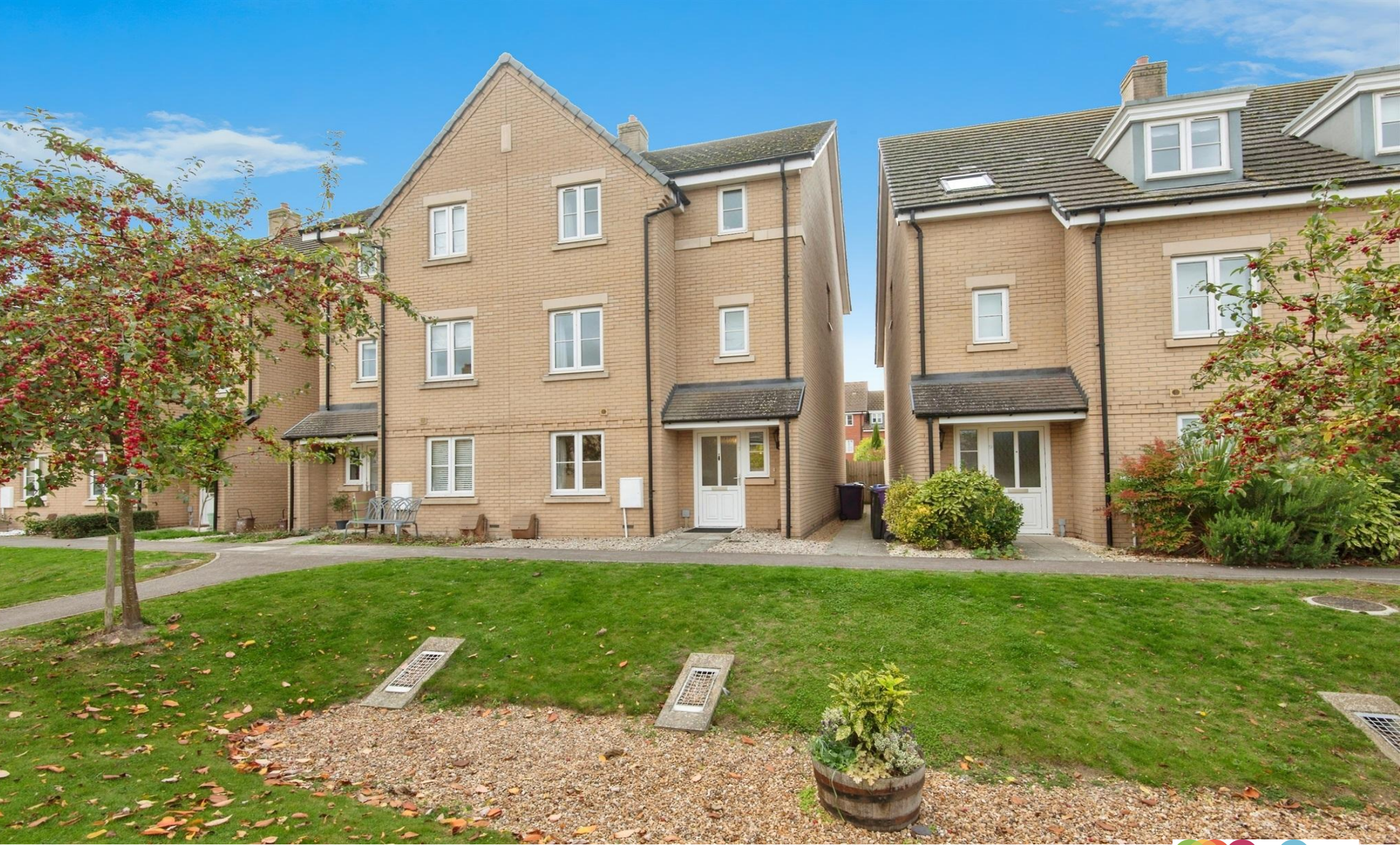
Grenfell Gardens, Royston, SG8 5FT
