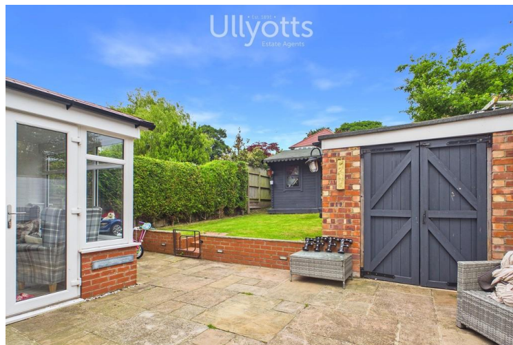
Patio and garage
