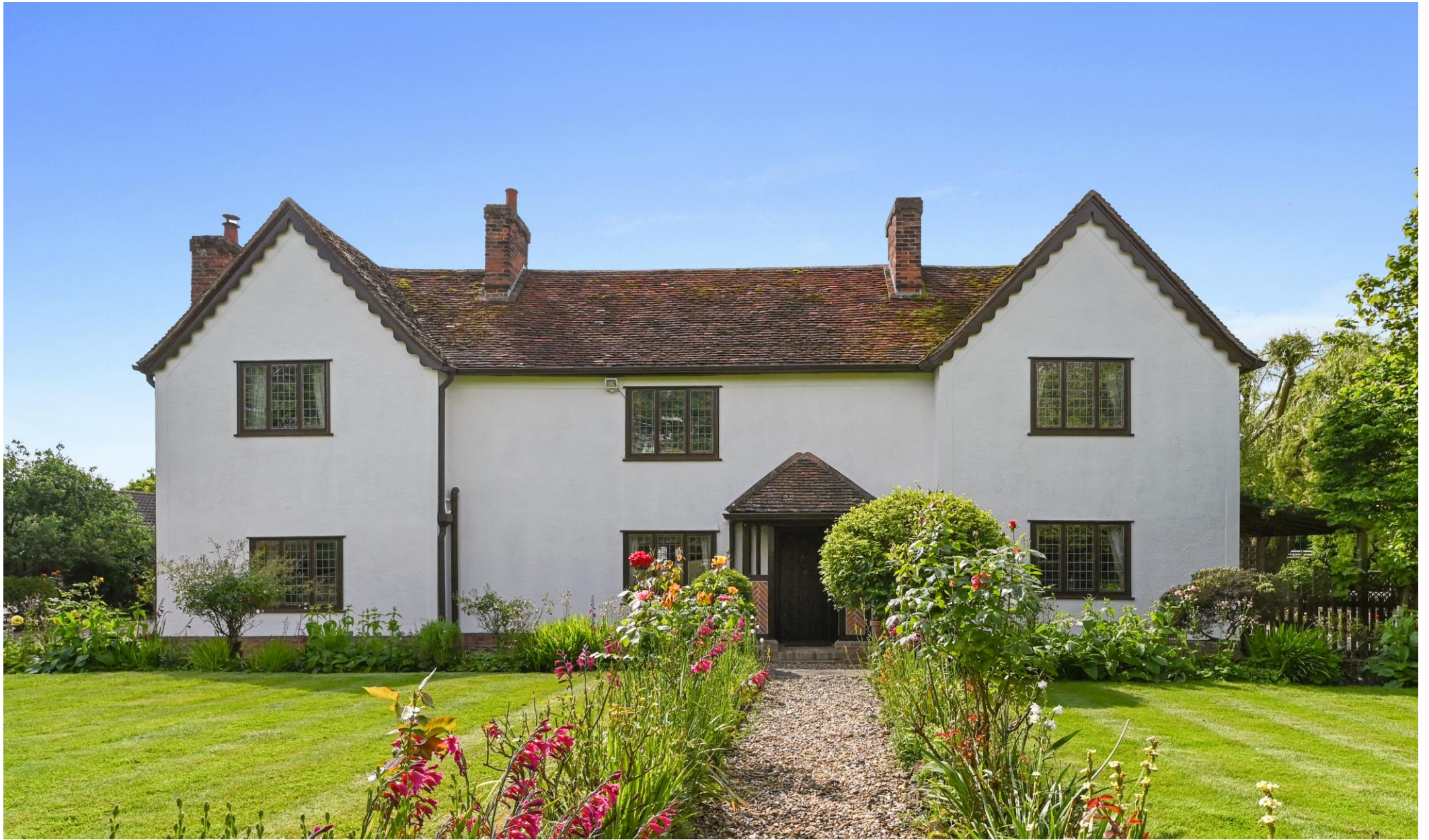
Godmans Farmhouse Coggeshall Road | Marks Tey | CO6 1LT
