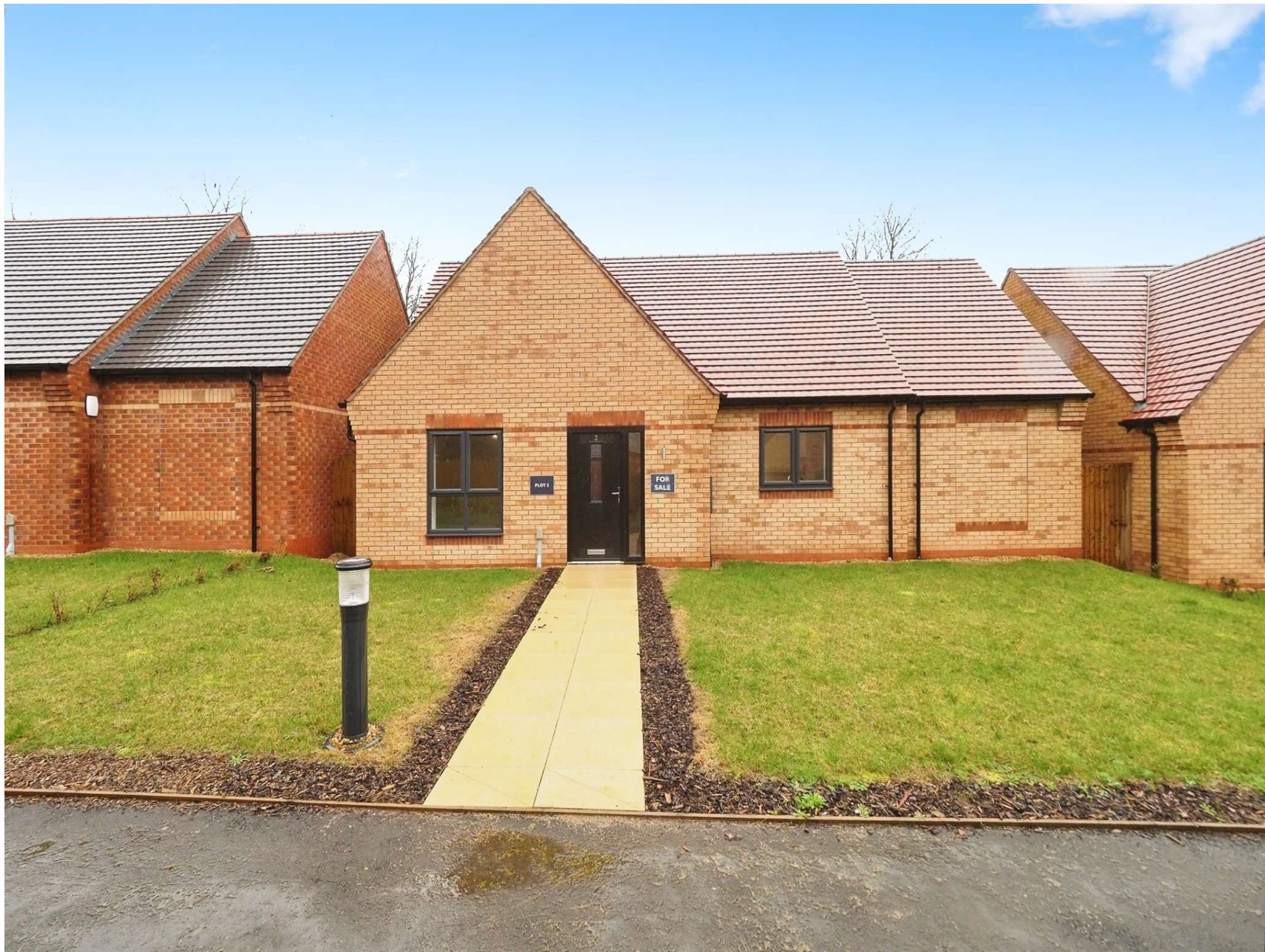
The Aspen Valley Lane, Mansfield NG18 2FP
