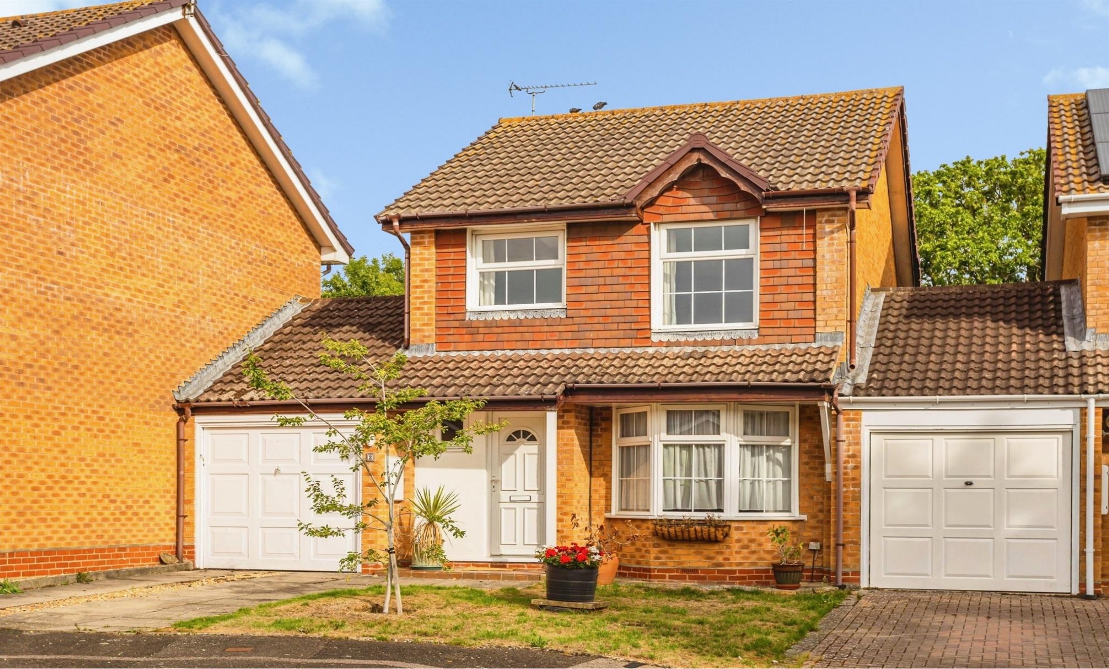
Langridge Way, Burgess Hill, RH15 8TN
