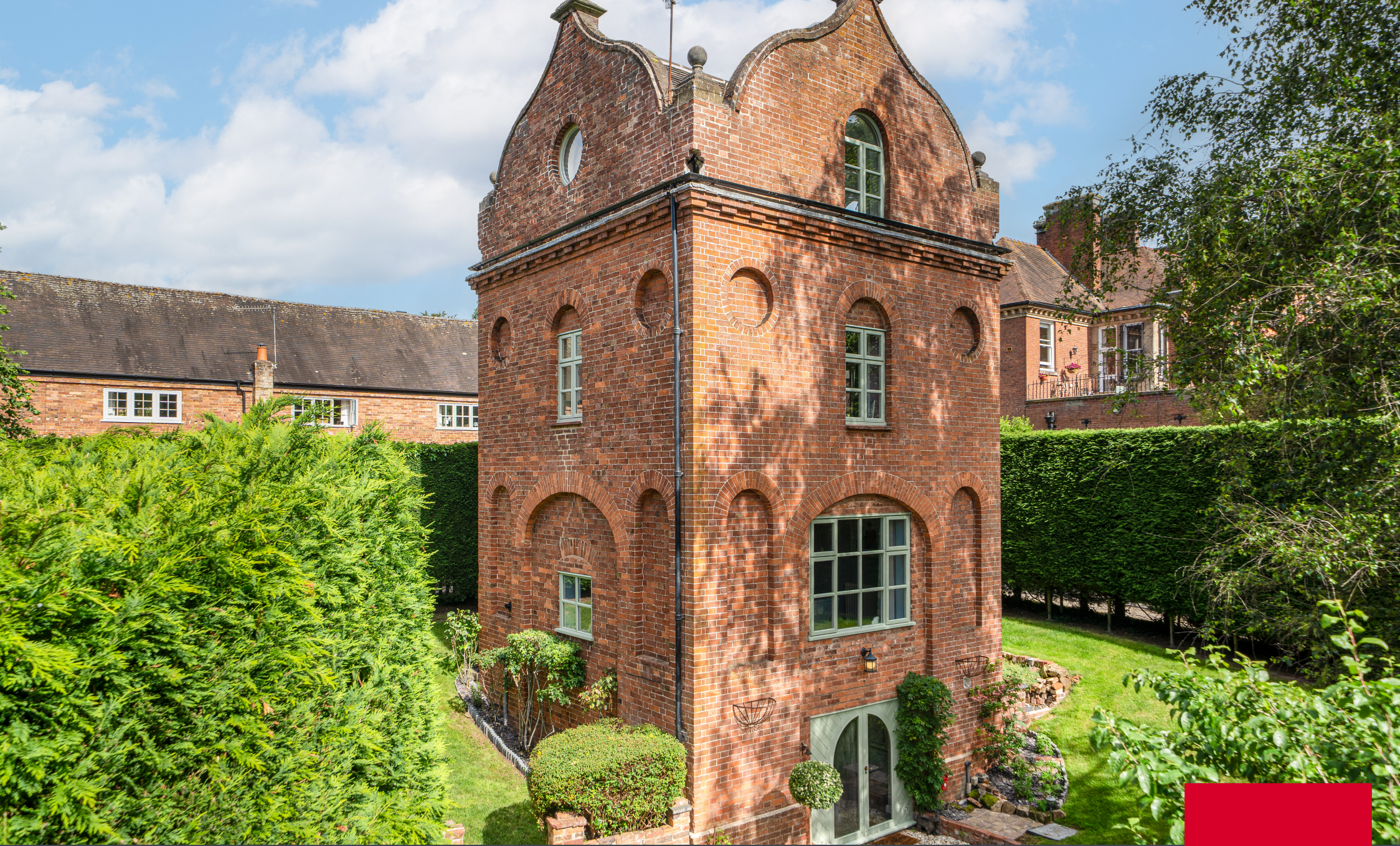
The Dovecote Wolverley Village, Wolverley
