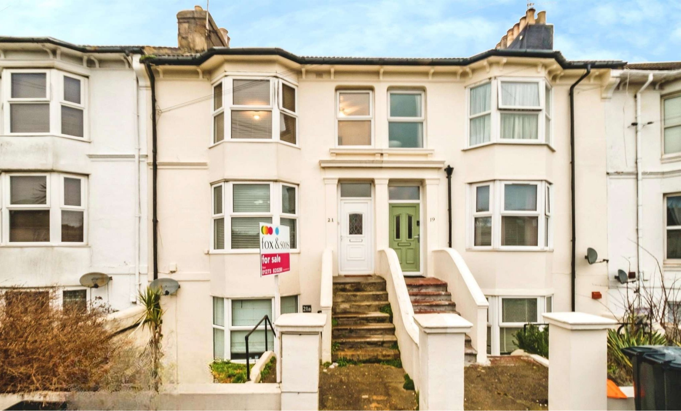
Shelldale Road, Portslade Brighton BN41 1LE
