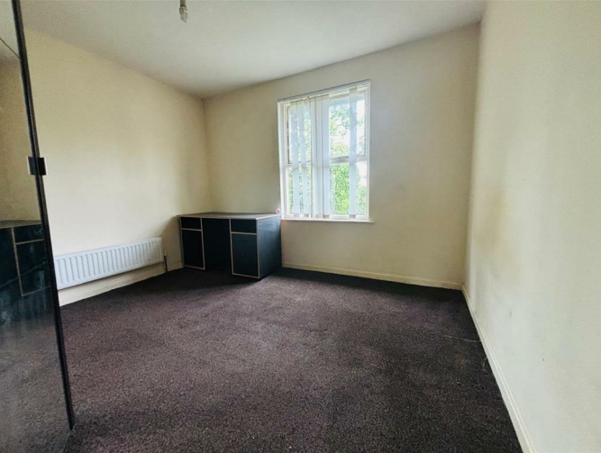
Double glazed window, central heating radiator
