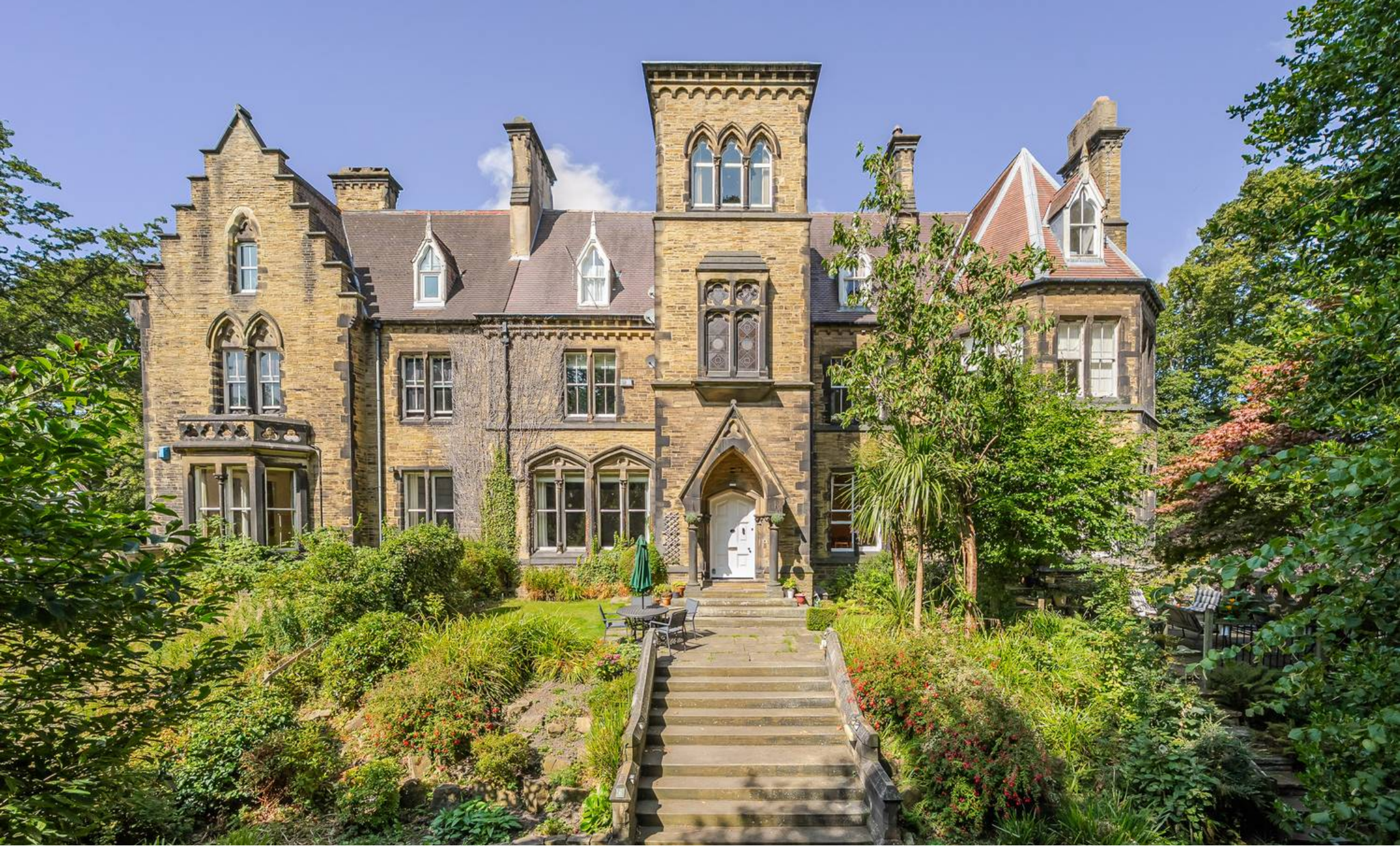
Grannum Lodge, Edgerton Road Huddersfield
