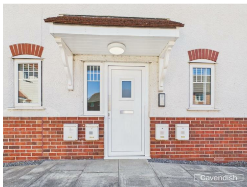
Communal entrance door with intercom entry system.
