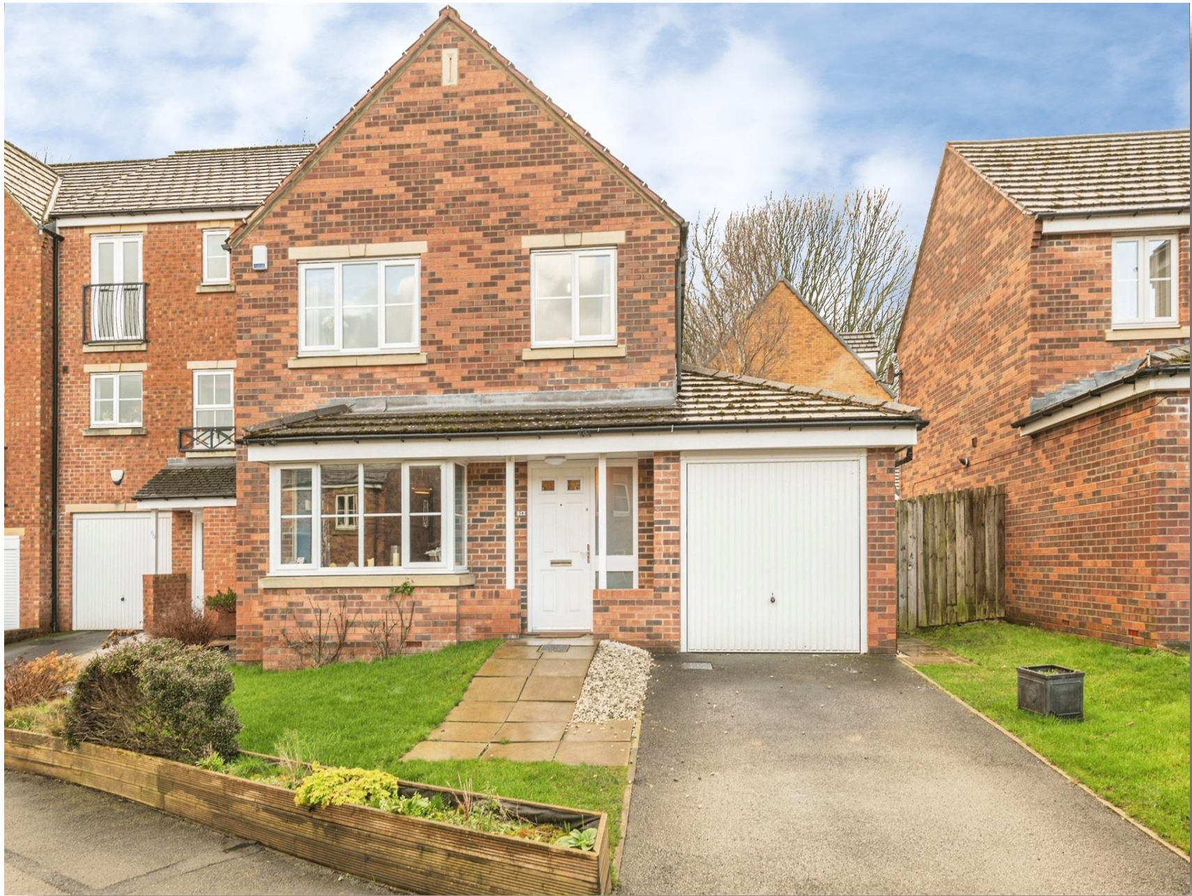
Hawthorn Lane, CLECKHEATON BD19 3TR
