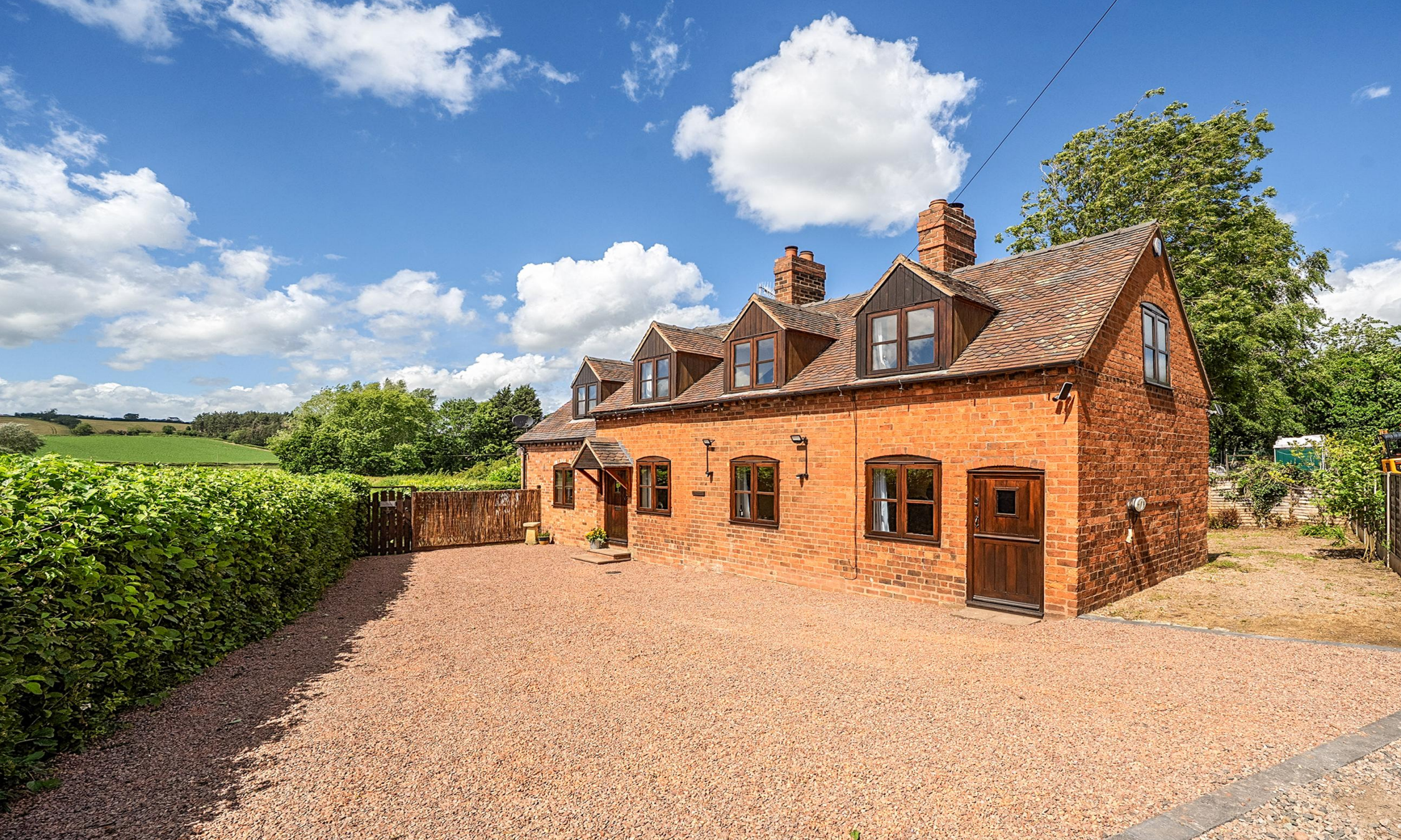
Lea Cottage, Dunley, Worcestershire
