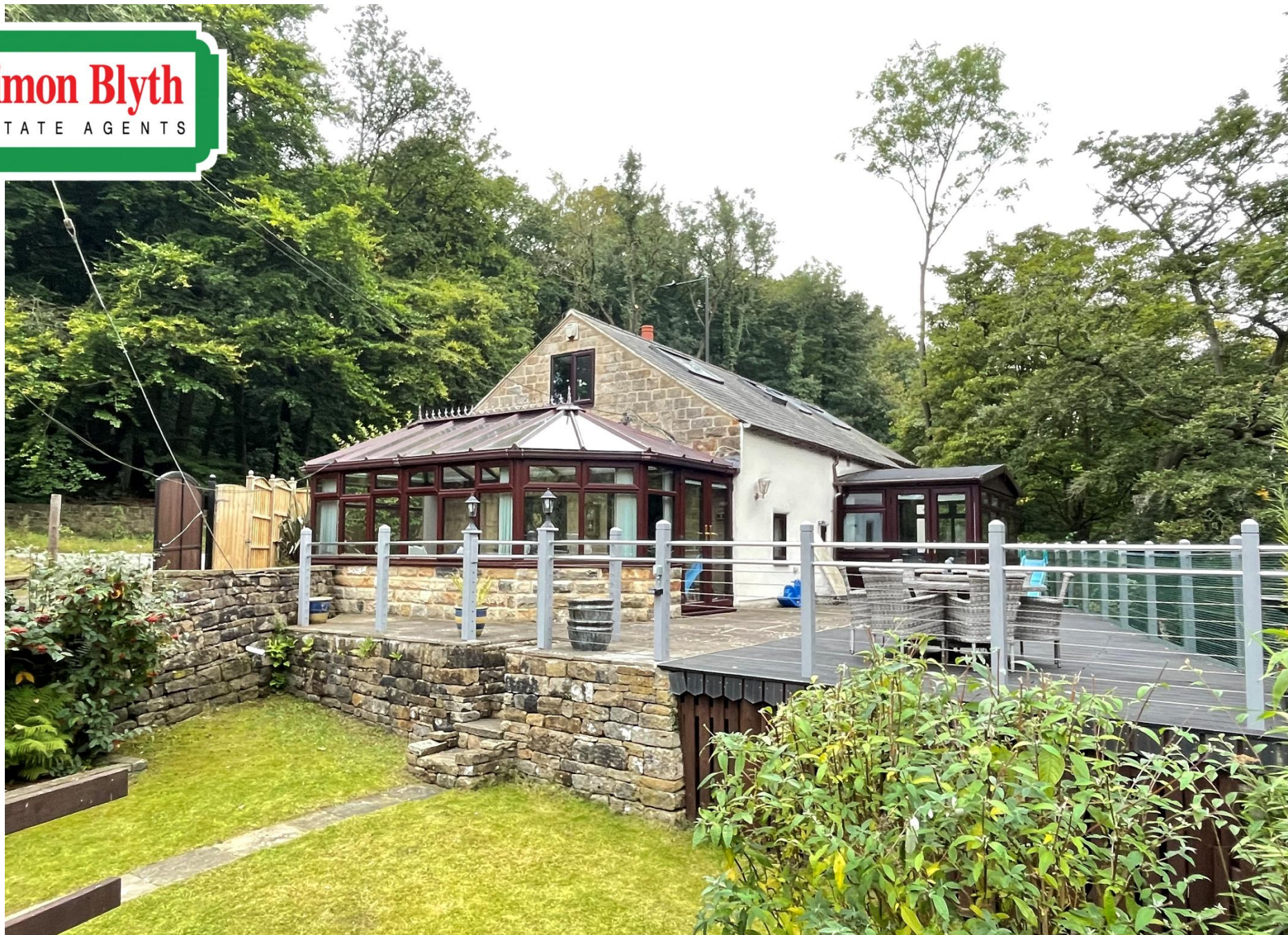
TOLL BAR COTTAGE, MIDDLEWOOD ROAD NORTH, S35 0HE
