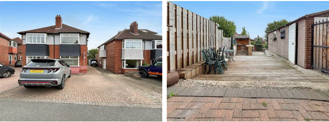
A block-paved area to the front and a driveway running to the side of the property provide useful off street parking for several family cars. The single garage is currently used as a workshop and has ample storage space, power and light.
