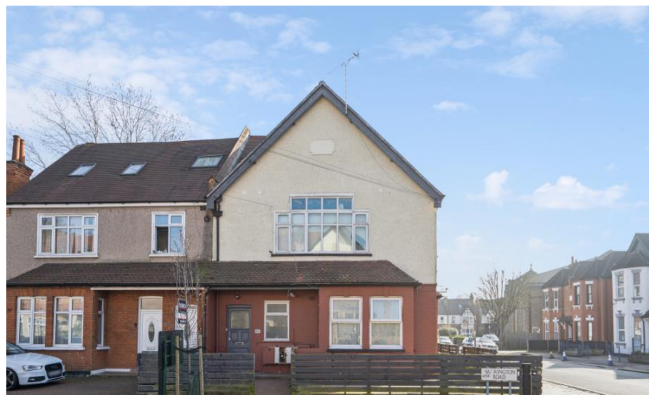
A recently refurbished first floor two bedroom duplex maisonette Warrington Road, Harrow, HA1 1SY
