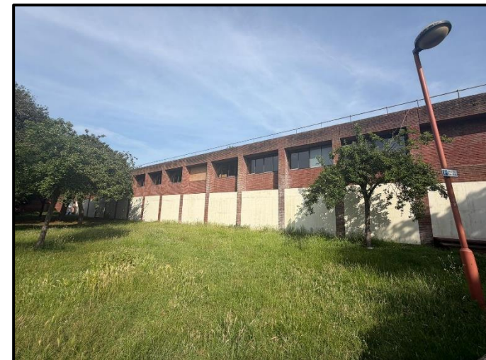
Existing Building (rear)
